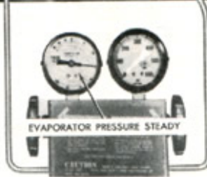
FIGURE 6—POA VALVE STUCK CLOSED
